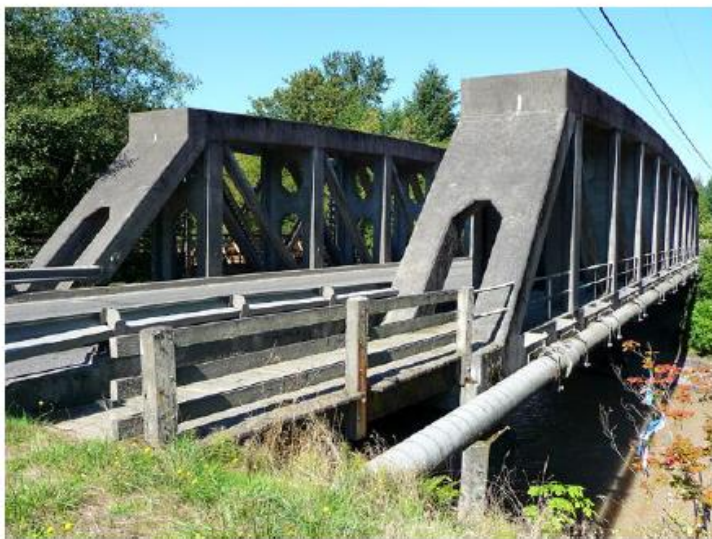
McMillin Bridge. WA : 1934.
