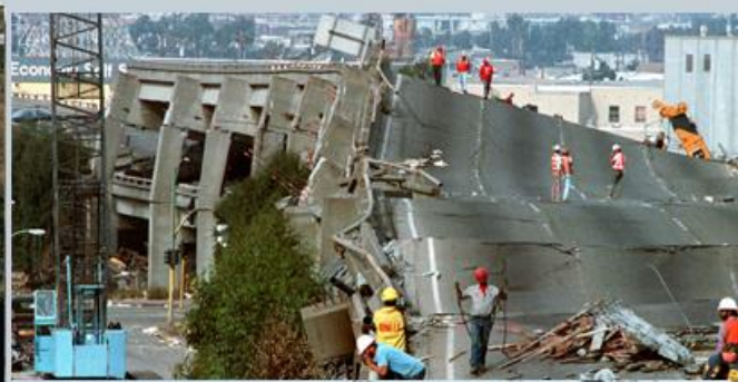
Cypress Street Viaduct Земљотрес Loma Prieta
