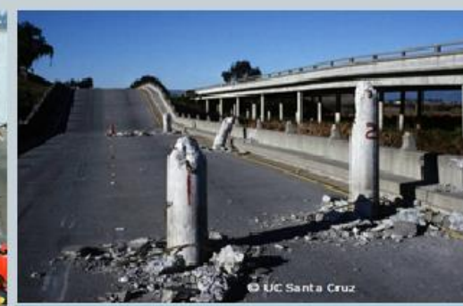
Struve Slough Bridge
