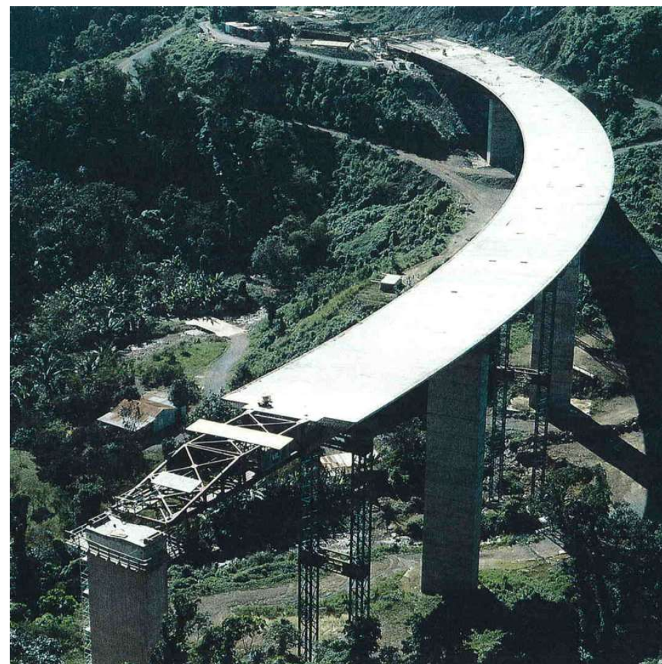
Caguanas river bridge, Porto Riko 1991.
