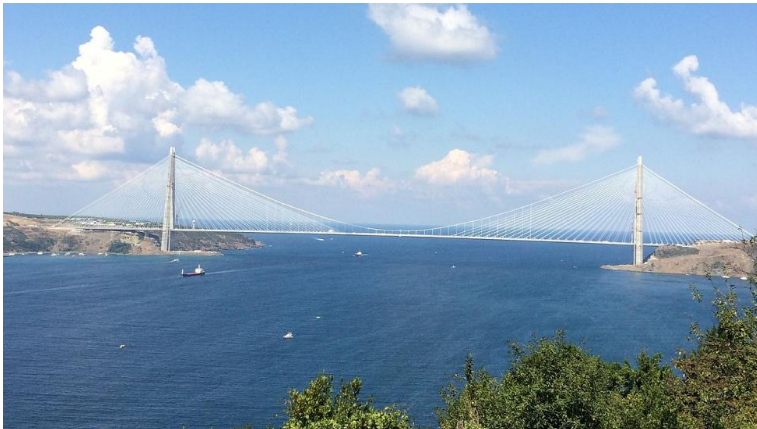
Yavuz Sultan Selim Bridge Raspon 1 408 m (2016.)
