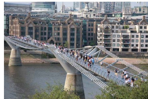
London Millennium Footbridge - 2000
